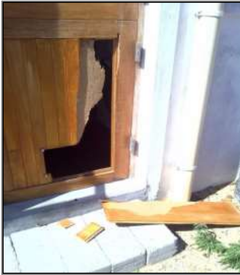
Figure.10. Photograph of damage to door caused DG6
